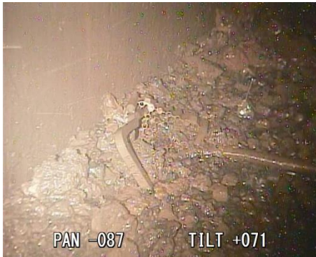
Photo: Near the pedestal inner wall at the Unit 2 PCV bottom
