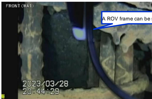
Photo 1: Concrete wall seen from the pedestal opening
